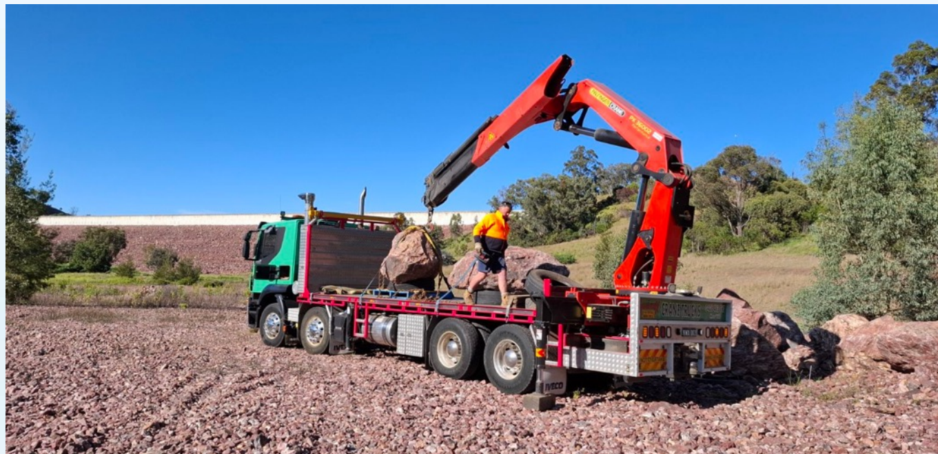
Uplift and loading of two chert boulders of approximately four tonnes. The white wall in the background is the top of Chaffey Dam. Image courtesy M. Smith.
