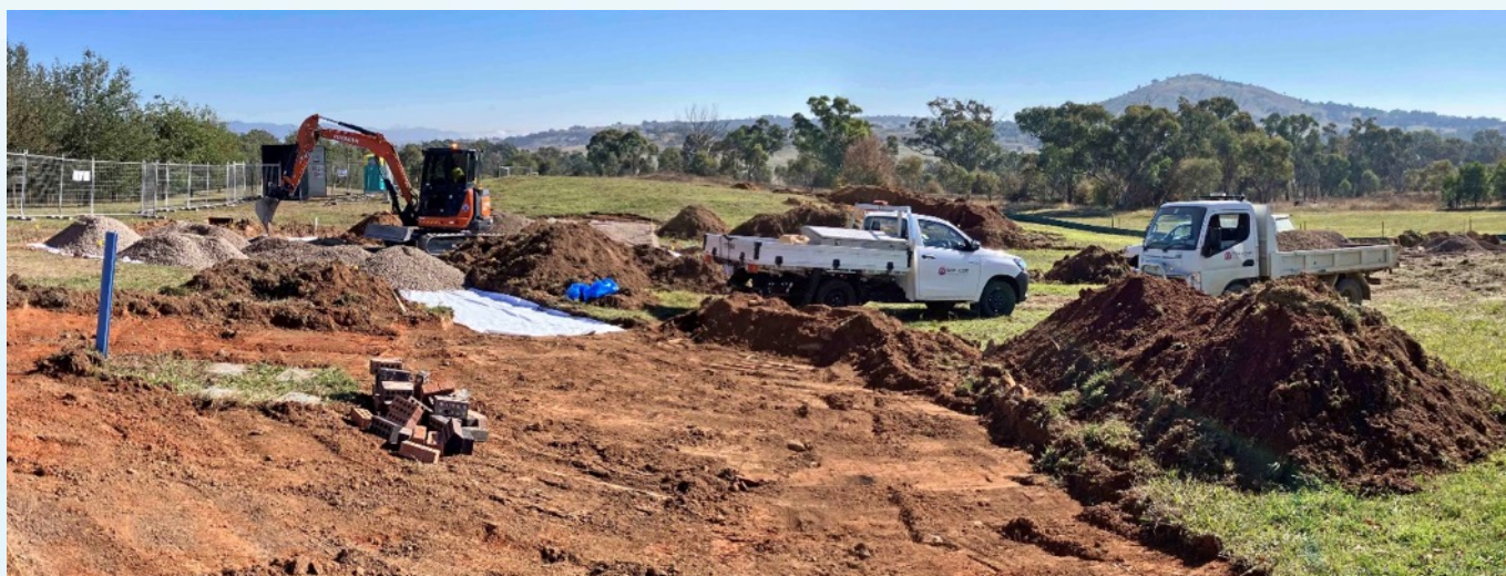
National Rock Garden Stage 1 path excavations, 17 May 2024. Image courtesy B. Pillans.
